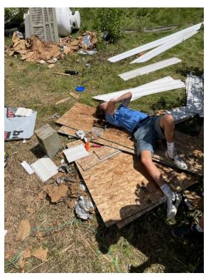
(If you don't know what this means ask anyone on this crew to explain it to you they are now professionals.) We then installed the new subfloor, installed a new plate and sistered the wall studs. We stabilized the structure of the home in this area and could then install the new base floor, reinstall the insulation, add exterior sheathing, Tyvek and put up
